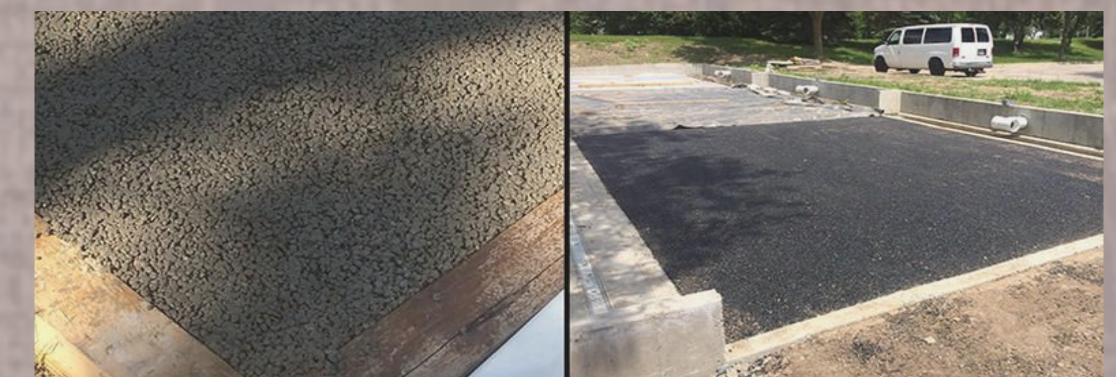
Figure 5a & 5b. Permeable concrete & asphalt that collect storm runoff water (Selbig 2018).
